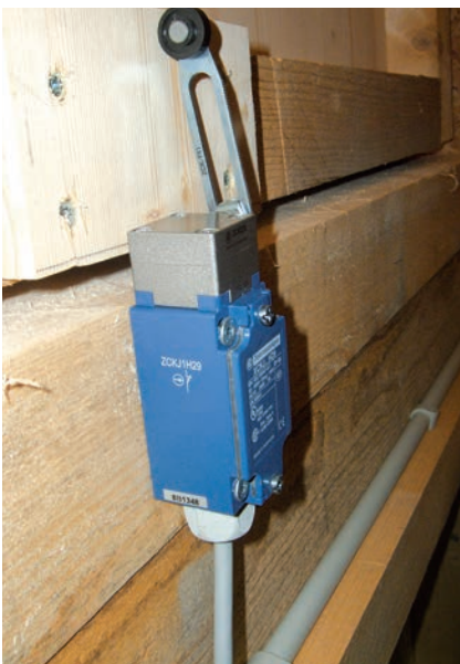
17 Air flap limit switch
