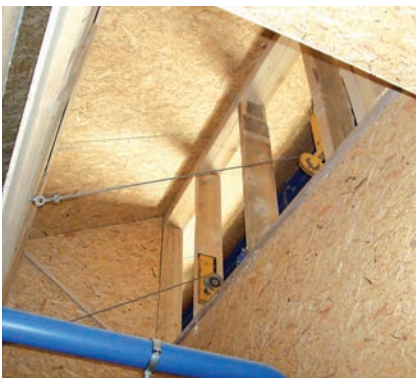
16 Recirculating air flap
