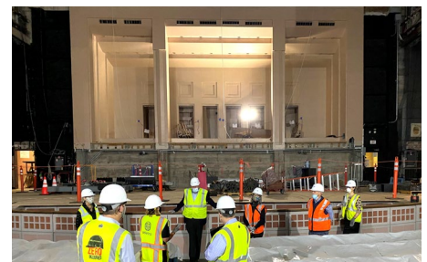
Installing Meyer Sound's Constellation Acoustic System
