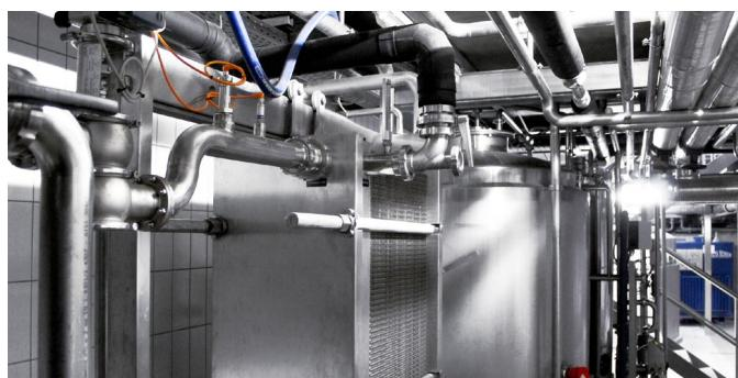
Keeping an eye on the process pressure assists in supervising the correct operation of the cooler. If particles or contamination disrupt the function, the pressure upstream of the cooler increases. In this case, the cooling system can be checked and, if required, cleaned to prevent damage.
