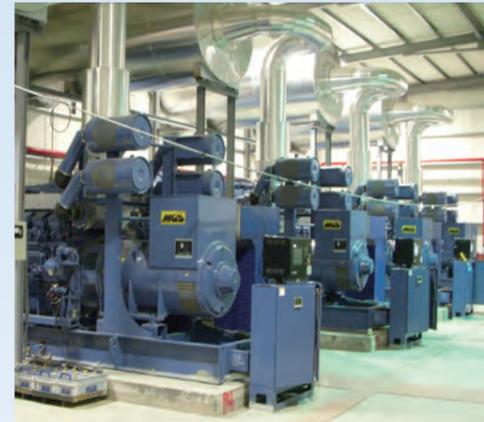
Whenever operating multiple generator sets in parallel, the prime mover and electrical systems should be protected to ensure stable load sharing characteristics, frequency stabilization, voltage stabilization and the synchronized closing of the circuit breaker.
